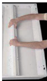
c) Remove ballast cover (lens removed)
